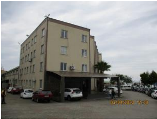
OVERVIEW OF THE FACILITY.JPG
