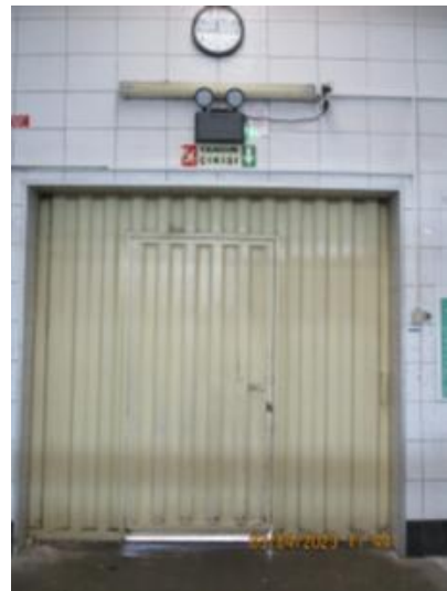
EMERGENCY EXIT DOOR.JPG
